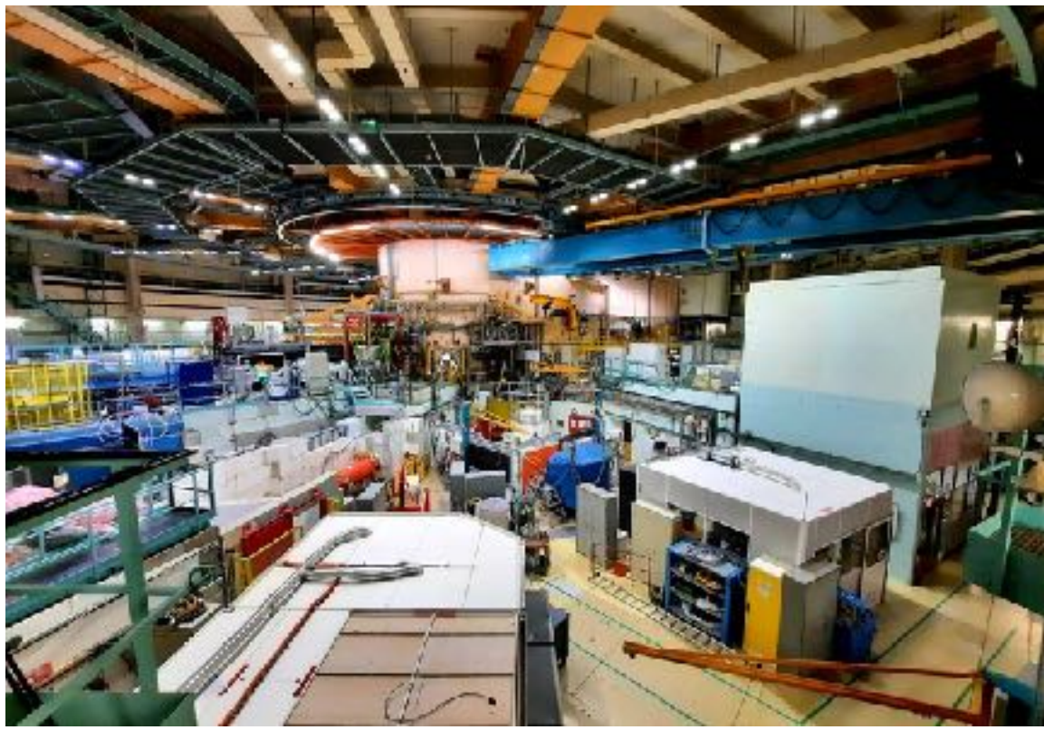
Inside the reactor hall of the Institut Laue-Langevin, Grenoble: the reactor core (rear) and the surrounding instrument floor, lined with the beamlines, shielding, and detectors used for neutron-scattering experiments.
